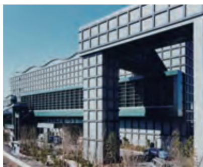
Noise control for a steam condenser intake: incineration plant
