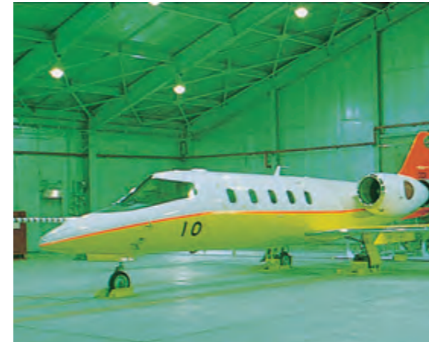
Noise control: hush house
