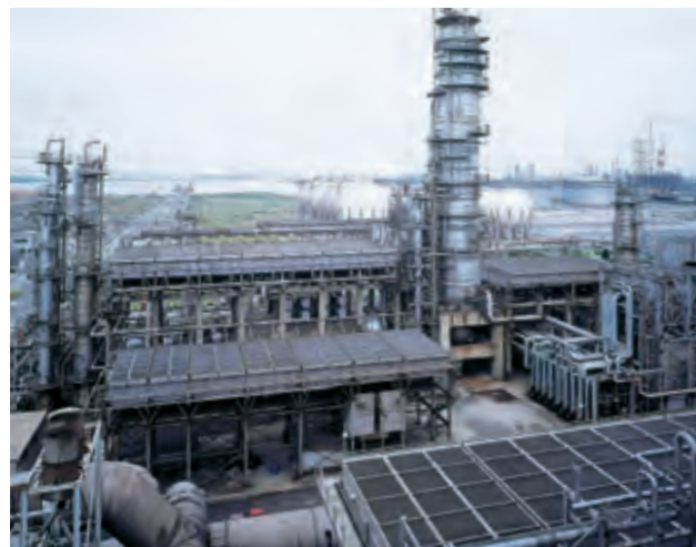
Air-Cooled Heat Exchanger installed in refineries and petrochemical plants
