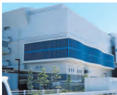
Noise control for a steam condenser intake: Nagoya City Inokoishi Incineration Plant
