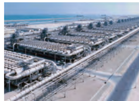
Multi-Stage Flash-Type Desalination Plant (MSF)
