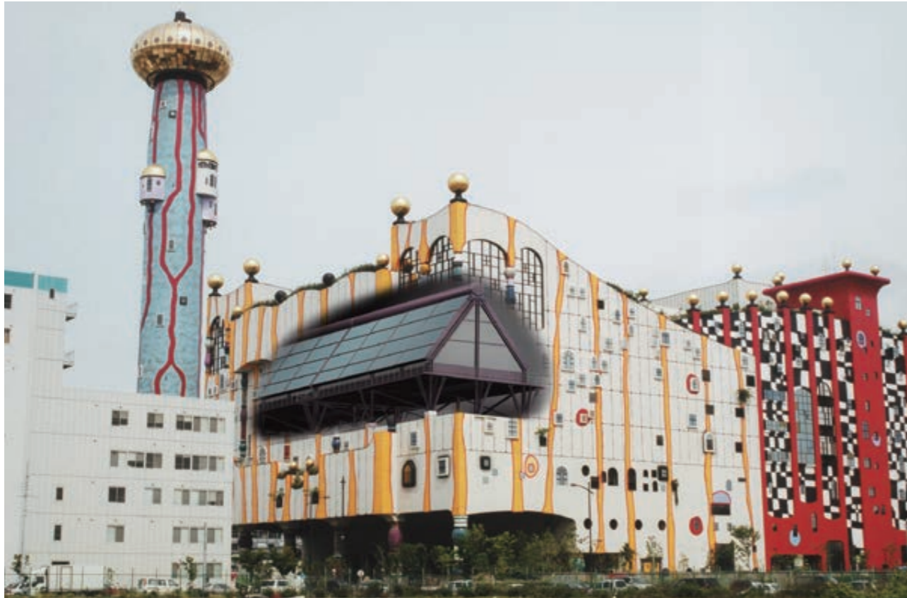
Air-Cooled Heat Exchanger installed in municipal incineration plants
