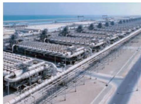
Multi-Stage Flash-Type Desalination Plant (MSF)
