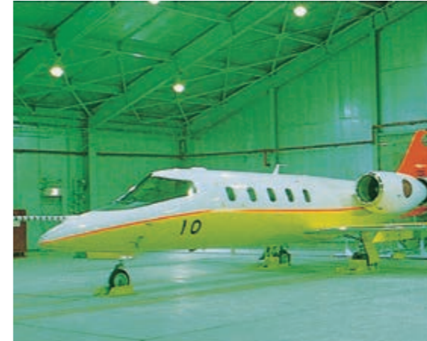
Noise control: hush house
