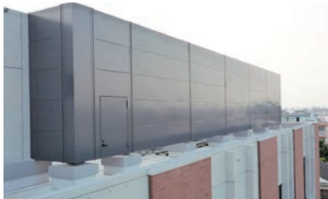
Noise control for an outdoor unit: data center
