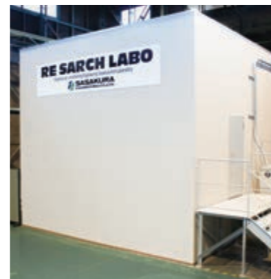
Hydronic heating and cooling radiation panel performance measuring room
