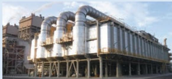
Reheat-Type Desalination Plant (MED)
