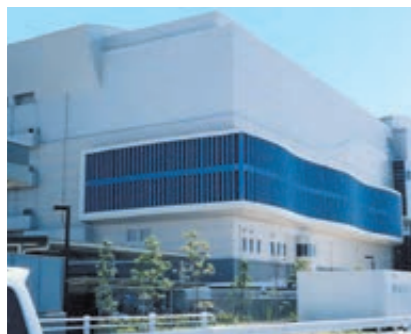
Noise control for a steam condenser intake: Nagoya City Inokoishi Incineration Plant
