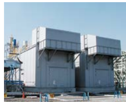
Noise control: gas engine enclosure
