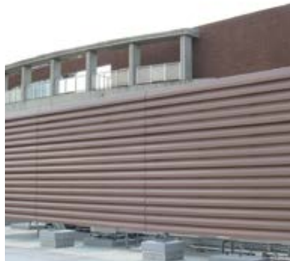
Noise control for an outdoor unit: facility in Osaka
