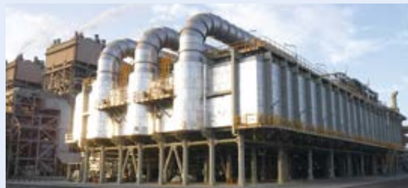
Reheat-Type Desalination Plant (MED)
