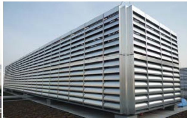
Noise control for an outdoor unit: data center
