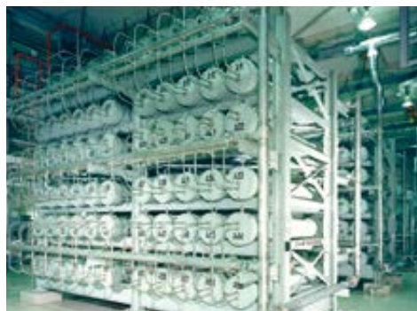
Reverse Osmosis Desalination Plant (RO)
