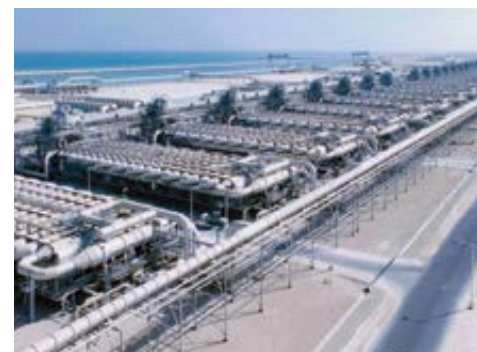
Multi-Stage Flash-Type Desalination Plant (MSF)
